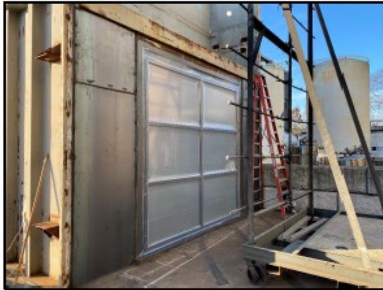
Photo No. 1 Exterior View During Static Air Infiltration Testing @ 1.57 psf & 6.24 psf
